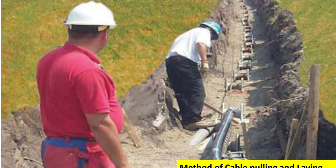
Method of Cable pulling and Laying
